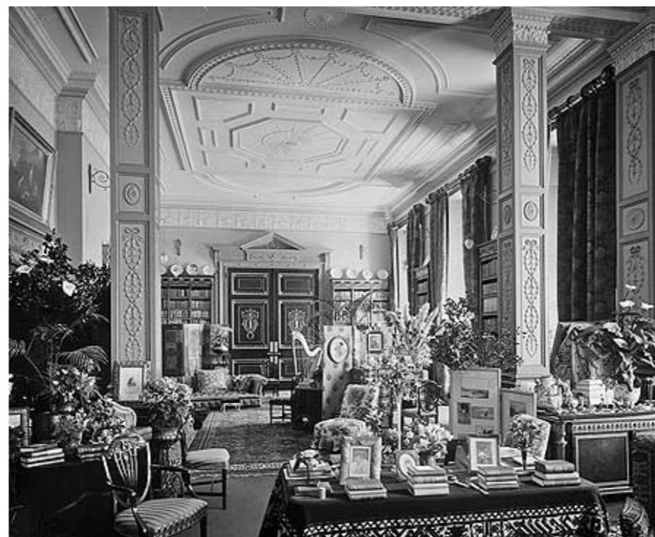
Figure A1.10 1892 - Library - Historic England archive Bedford Lemere
