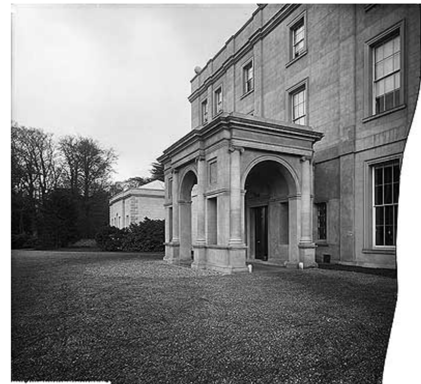
Figure A1.20 1892 Porte cochere – Historic England archive
