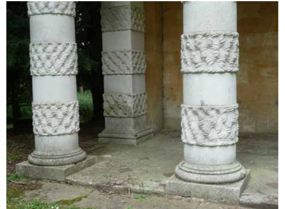
Figure 4.8 Detail of rustication on columns.
