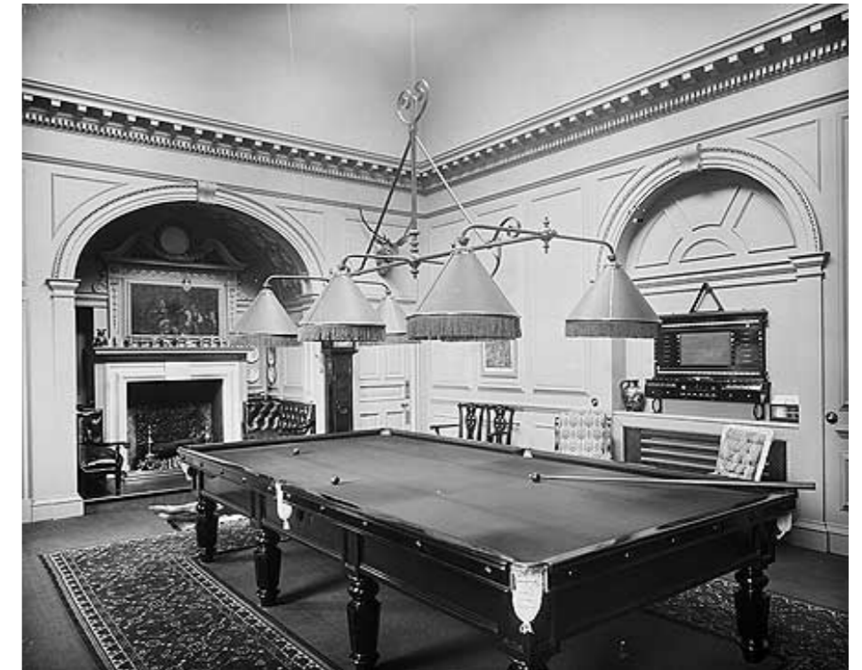
Figure A1.11 1892 Billiard Room - Historic England archive Bedford Lemere - later blue room
