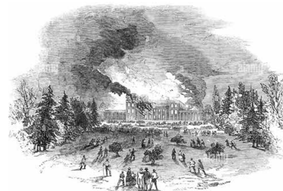
Figure 3.4 An image that appeared in the Illustrated London News of 1850 "Destruction of House by Fire"
