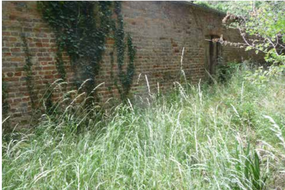
Figure 4.17 The east kitchen garden wall, mostly of 18th-century date but the top ten courses or so of 19th-century date. It is in fairly good repair.
