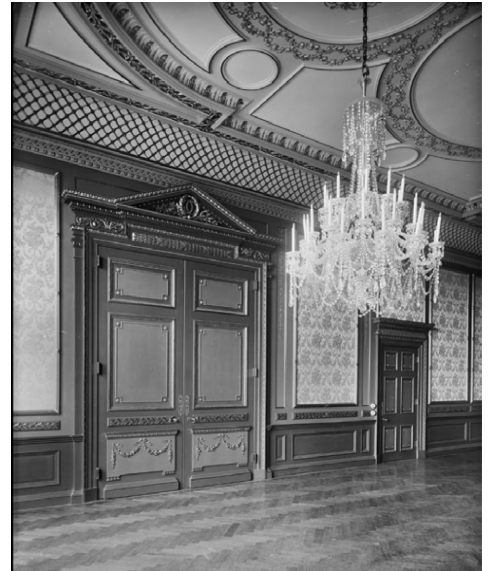
Figure A1.15 1892 Doors in Dining Room – Historic England archive
