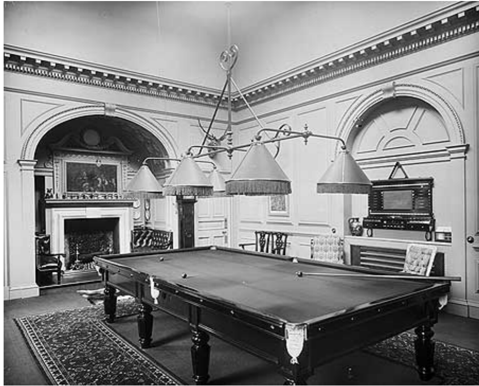
Figure A3.1 1892_billiard room_HE archive_BedfordLemere_later blue room
