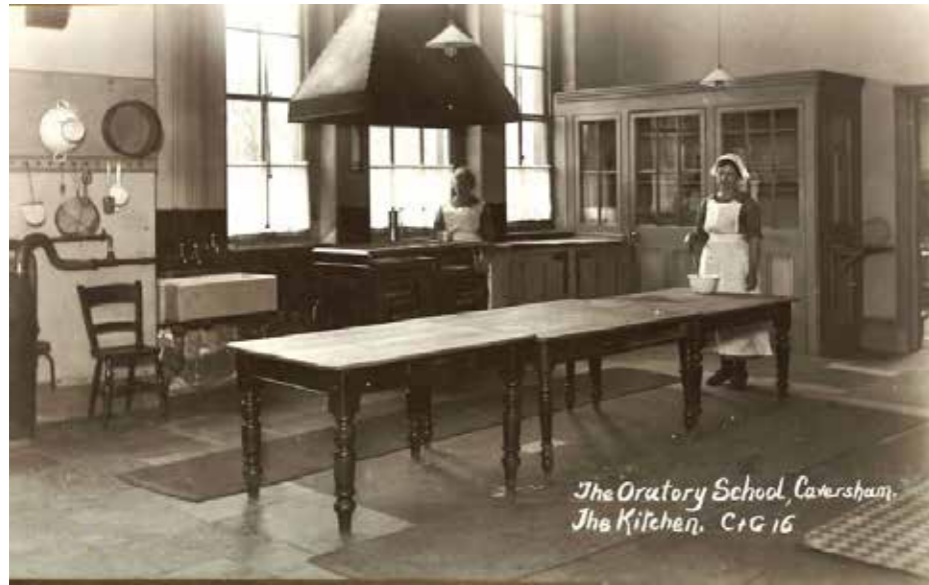
Figure A1.79 1930s Oratory School archive kitchen
