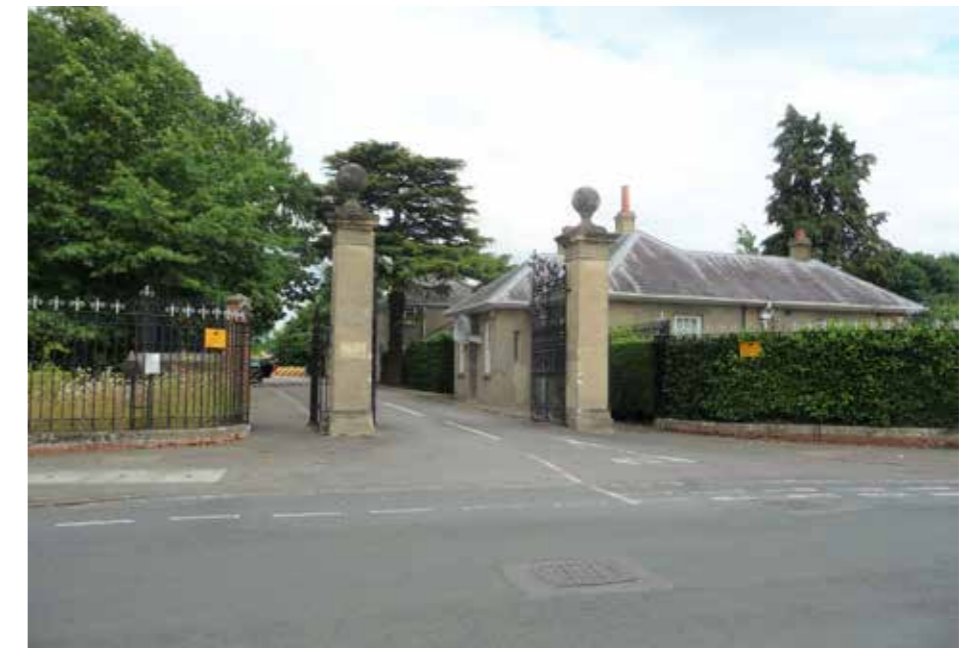
Figure 4.1 The north-west entrance lodge.
