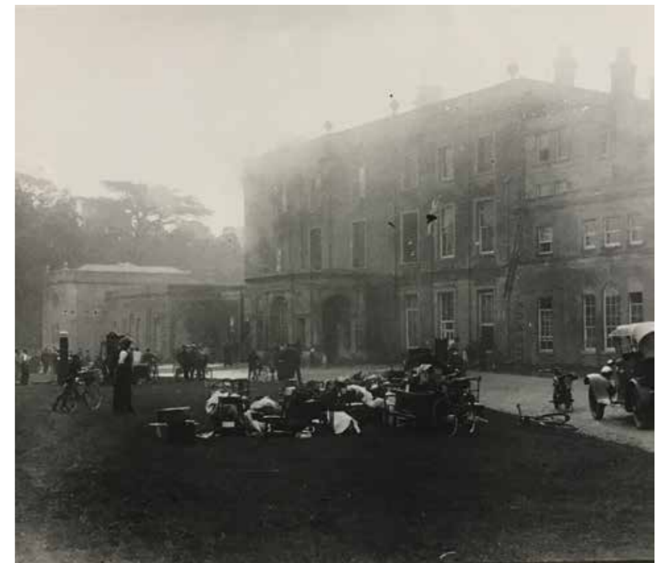
Figure A1.63 1920s ground floor colonnade
