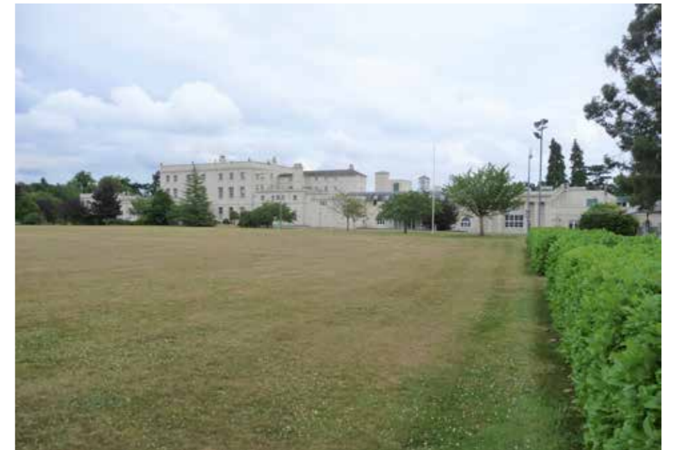
Figure 4.11 Looking north-east to the house across the third of the terraces.
