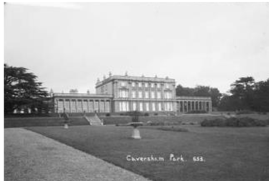
Figure 3.14 The exterior of Caversham Park, taken by photographer Phillip Osbourne between 1905 and the mid-1930s, Museum of English Rural Life, Reading
