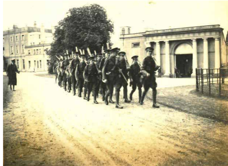
Figure A1.69 1923 Oratory school archive off to camp
