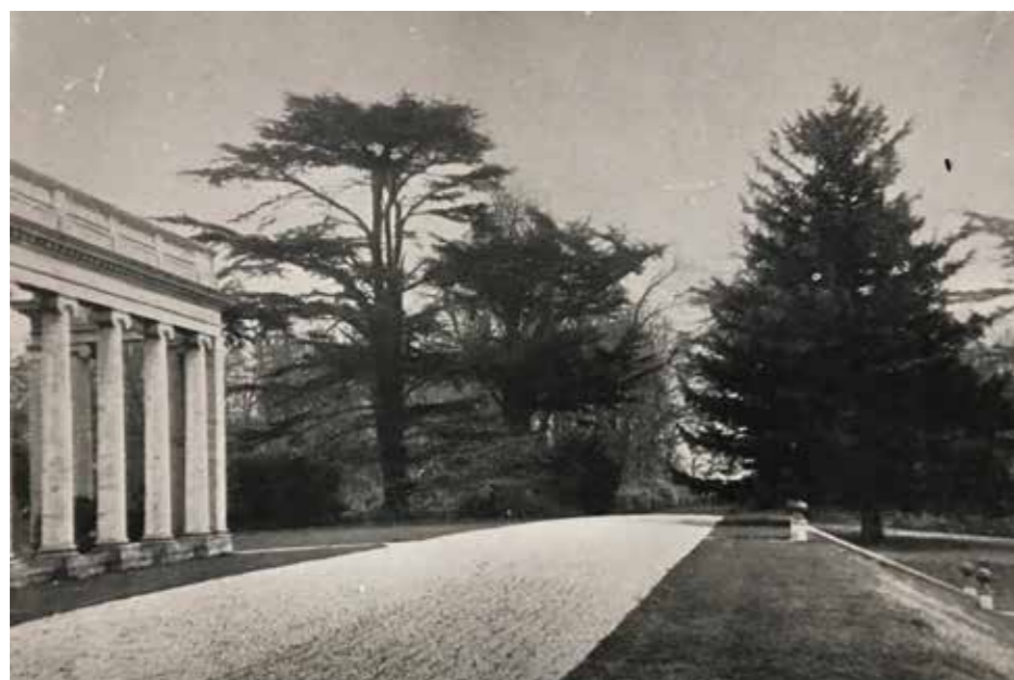
Figure 3.9 The Terrace in 1897, Berkshire Record Office
